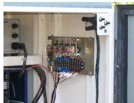
Figure 3: Relay board installed in signal cabinet to provide logic for TSP loops.
