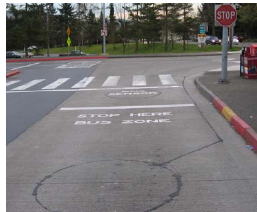
Figure 5: Pavement markings installed over TSP loops near the southbound bus stop.
